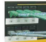
Patch Panel Identification
