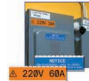
Electrical Panel Identification
